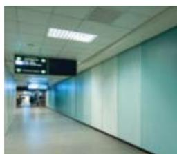
In 1989, contractors installed 16 200 m<sup>2</sup> of Formica SolidCore in seven different shades of the aptly named 'Sky Blue' colour series. Today, despite the twenty million people that pass through the airport annually, not a single panel has required replacing.
